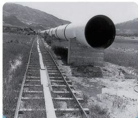
接收深圳水庫供水的大型水管，直徑約48吋。 A large pipeline with a diameter of about 48 inches for the reception of water from Shenzhen Reservoir.
